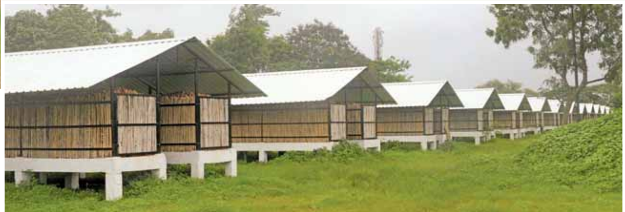
(Above): NAFED's unique ventilated structures for storing onions at Pimpalgaon, Nasik. (Below): Chawls are multi-level structures made from bamboo and secured with iron net
